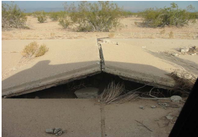
In addition to being a serious safety issue, the pavement at this airport inspected by the FAA needs obvious repair. Letting airport pavement deteriorate to this level is inconsistent with the sponsor’s grant assurances. (Photo: FAA)
