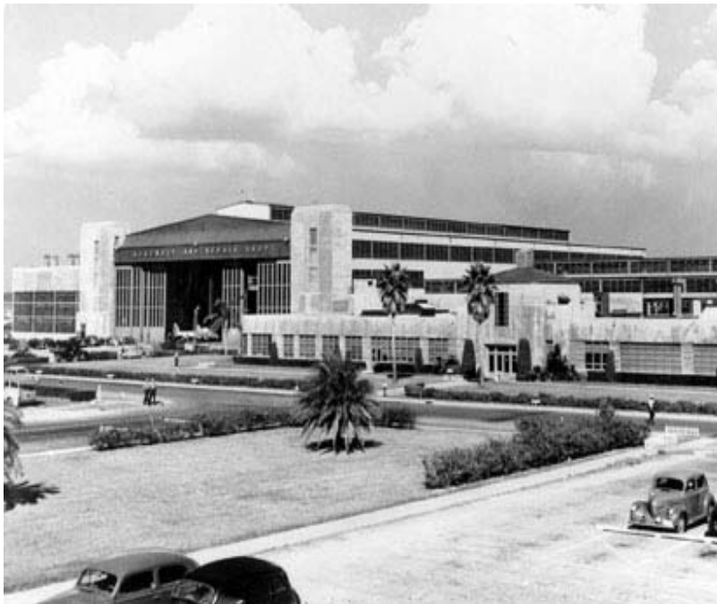
Following World War II, under the provisions of the Surplus Property Act of 1944 (section 13(g)) (as amended by 49 U.S.C. §§ 47151-47153), large numbers of military installations were conveyed without monetary consideration to public agencies. (Photo: US Navy)
