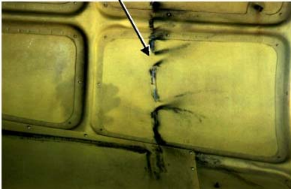
FIGURE 19-22. GAPS IN BAFFLE SEAL
